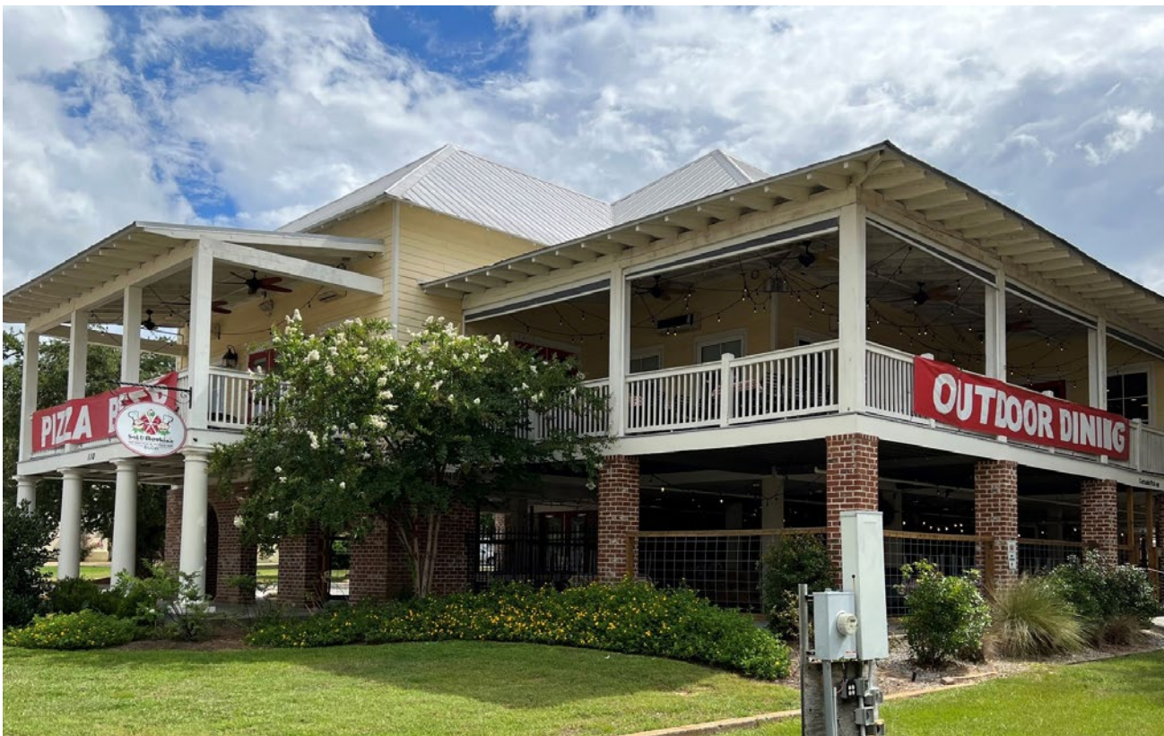
Example of a Commercial/Restaurant Use in a Floodplain with Parking on the Lower Level
