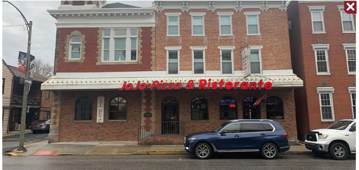
Bad example showing smaller windows that were used to replace original storefront windows.
