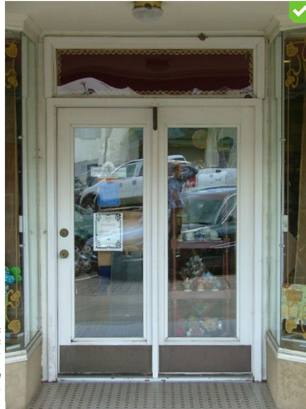
The material, detailing, and lack of transparency in these doors are inappropriate replacement solutions.
