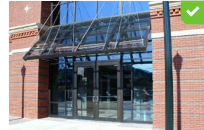
Metal and glass canopies interpret the historic role of a canvas awning and clarify entry on this new building.
