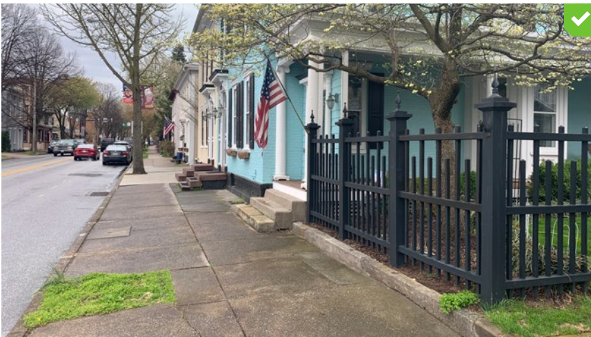
Good examples of fence and wall elements that define public and private spaces while allowing visibility between spaces. Note that the fences and wall elements are more ornamental in response to the traditional adjacent architecture.
