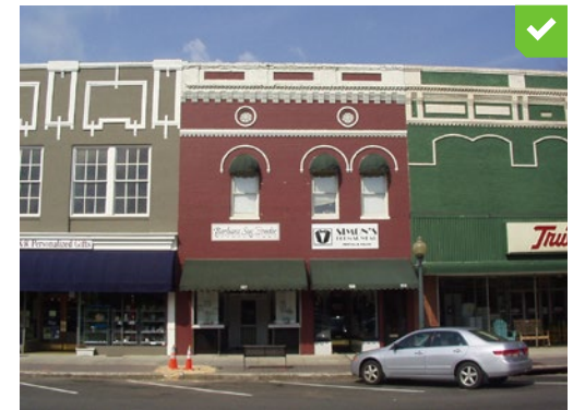
Both variety and uniformity were attained in the treatment of the roof line of these three buildings.
