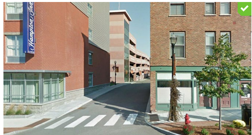
Examples of parking structures constructed behind uses along the main commercial street.
