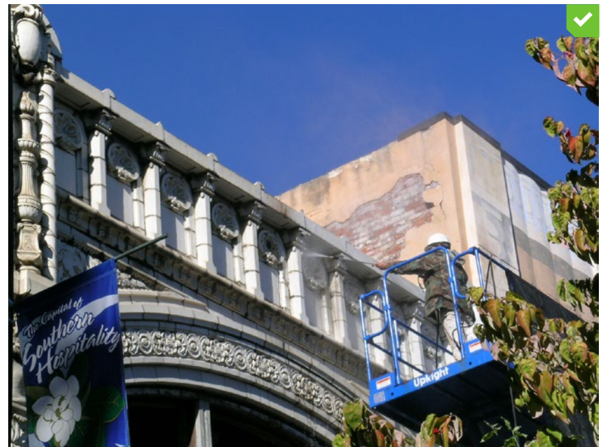
Terracotta cornice cleaning via a low-pressure water wash and mild detergent.
