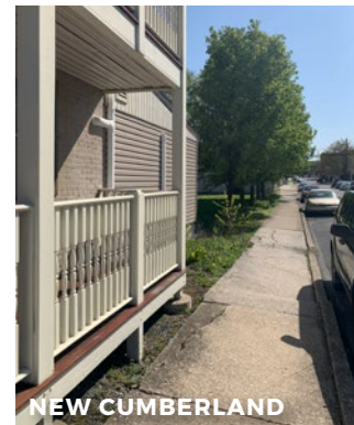
Crawl spaces under porches should remain open or covered with a recessed screen to maintain ventilation.
