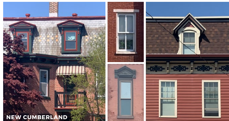
Many windows throughout New Cumberland Borough are quite modest; though some buildings follow a tradition of historic windows with ornate trim and window hoods.
