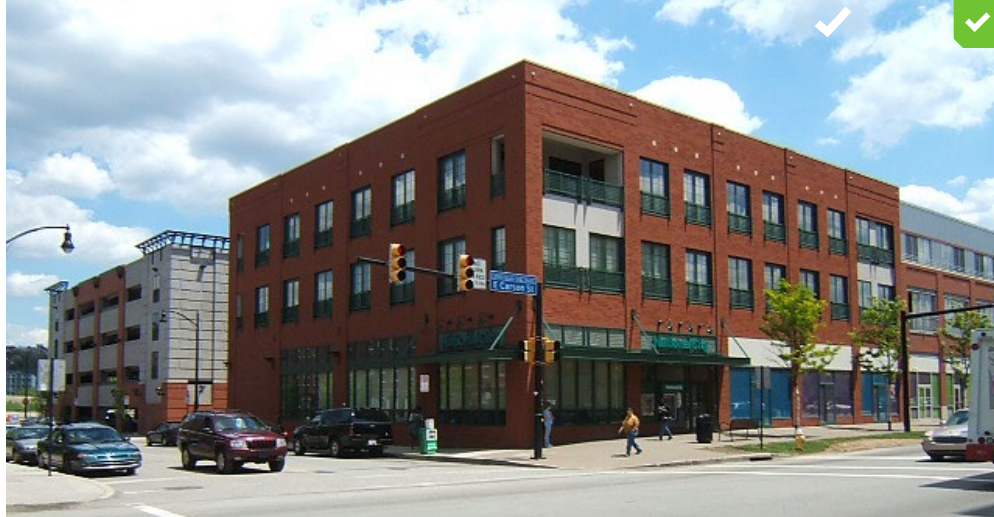
The storefront windows on the first level and regularly spaced punch windows on the upper floors demonstrate how a new commercial building can reflect traditional early Twentieth Century commercial buildings.
