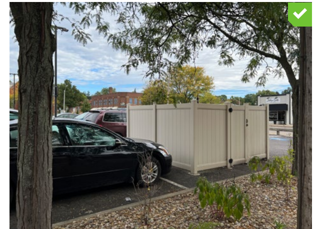
Example of a simple dumpster screening where a rear alley joins a parking area.
