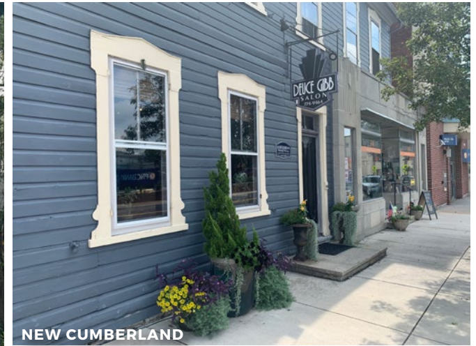
Wood frame is a common historic building material; however, it has often been covered or replaced with aluminum or vinyl siding.
