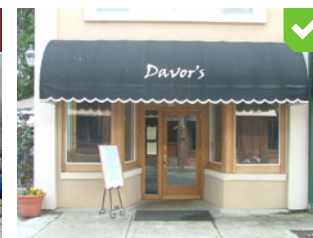
One way to deal with the transom area is to conceal it with an awning. All the other elements of the traditional storefront are dealt with appropriately in this example.
