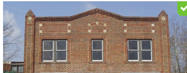
The triangular treatment at the center of the roof line creates interest and delineates entry. The upper floor details such as pre-cast tiles and recessed panels above the windows creates interest at the second floor.
