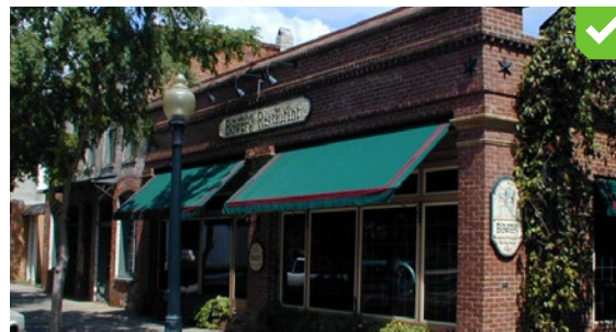
Perfectly executed awning installation.
