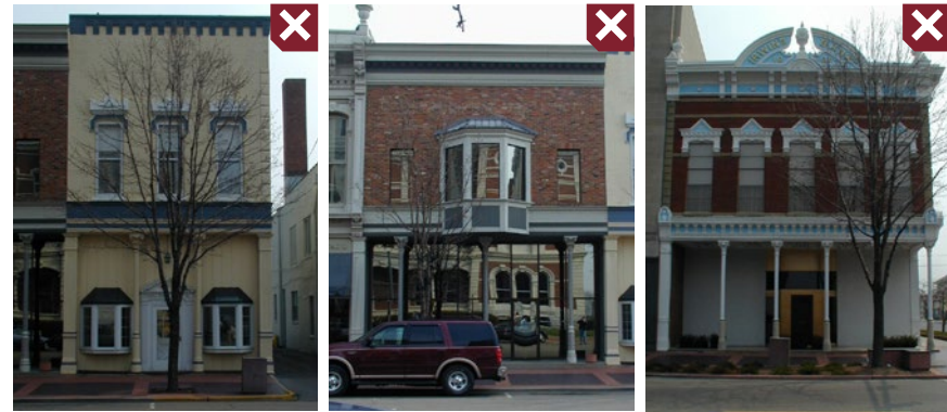
Examples of inappropriate storefront renovations & replacements.
