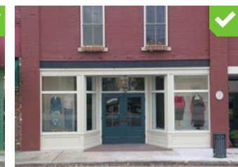
Good example of storefront renovation utilizing new materials adhering to traditional storefront composition.
