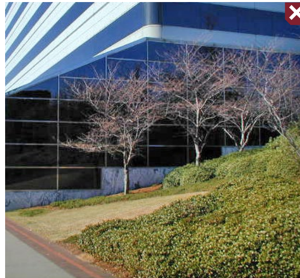
Blank wall at pedestrian level is unappealing. Scale & proportion of upper floor windows are incompatible with surroundings.
