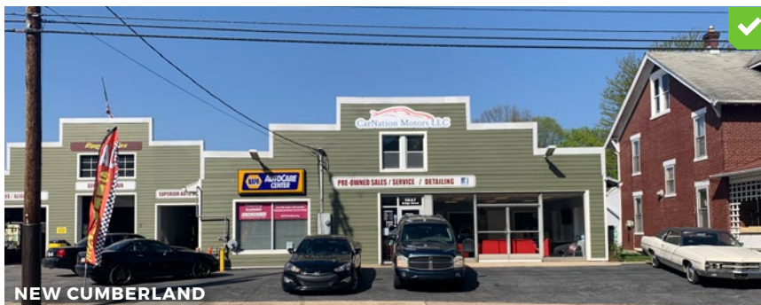
Good example of an automotive use with an attractive façade.
