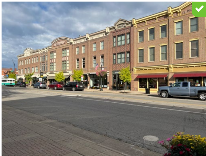
The façade of this new infill building that covers most of a block length was articulated so that it appears to be a series of individual buildings that match the scale of nearby historic buildings.
