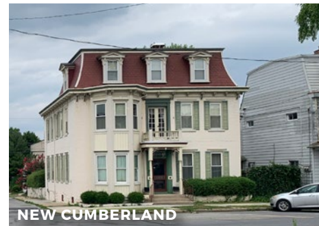
Mansard roofs are on many buildings throughout downtown.
