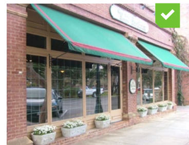
The preservation of the existing brick on this building relates it to the entire downtown area.
