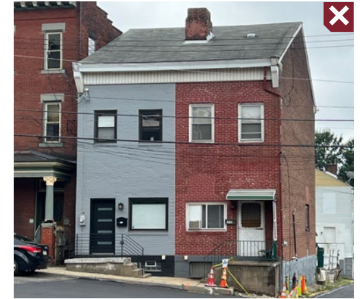
Replacement of the original windows on these two residences clearly results in an ill-proportioned façade. Note the bricked-over original window openings.
