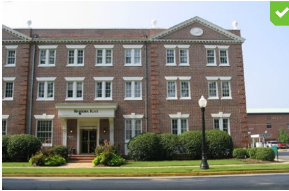
Large building sub-divided into bays with clear hierarchy and delineation of entry.
