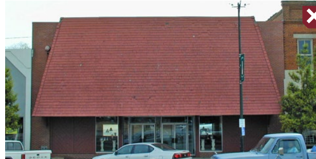
The roof form becomes the dominant element of this façade and is incompatible with its surroundings.
