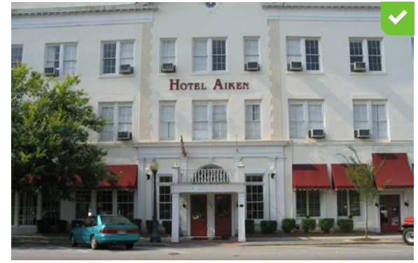
Long building sub-divided into bays with clear hierarchy and delineation of entry.
