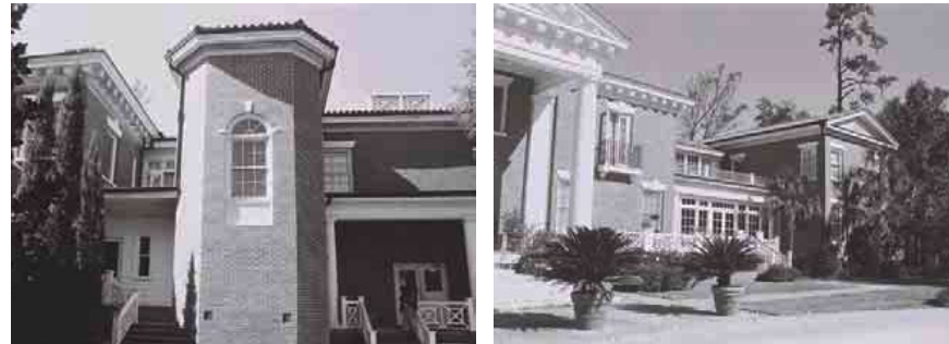
Built in the early 1900s, this residence was enlarged considerably for use as a hotel. Both rear and side additions were made for the new use. While the brick and roofing of the additions match that of the old structure, the detailing is less elaborate. The form of the original house, which is still dominant, is evident.
