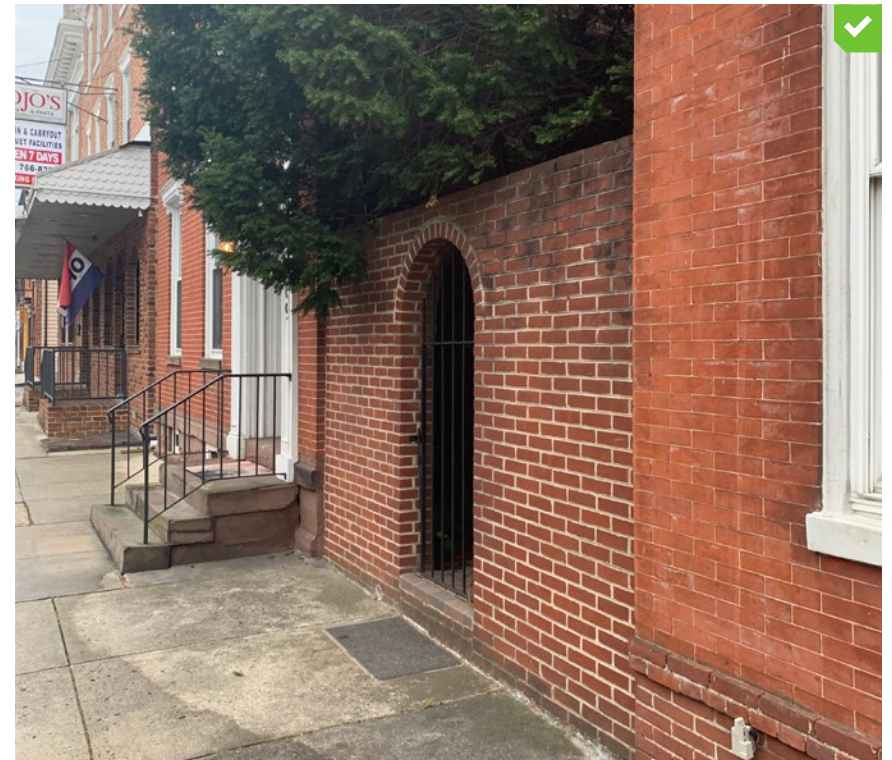
Good example of a tall wall that uses the same materials of the adjacent building and provides more privacy while still including transparency through the gate.
