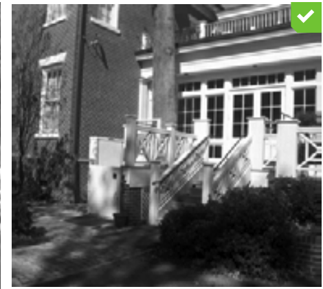
The wheelchair lift provides access near the front entrance and eliminated the need for a ramp. Such lifts are effective for three-to-ten foot changes in elevation.
