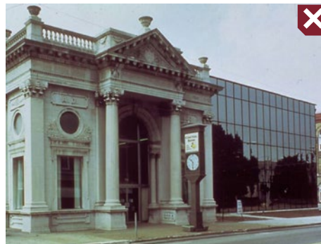
Negative example of a property satisfying the criteria to “be distinct” from the original structure, but failing miserably to “be compatible” with the original structure and its surroundings.
