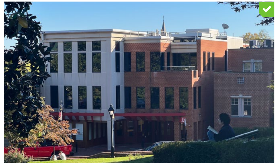
Examples of new commercial/mixed-use infill construction compatible with traditional downtown character.
