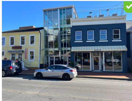
Example of new addition to make upper floors accessible with an elevator. The addition respects the essential form and integrity of the two historic structures it connects.
