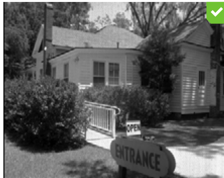
This appropriate handicapped ramp is easy to locate from the off-street parking area and is inconspicuous from the street.
