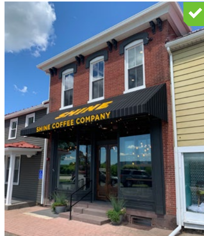
Good example of an awning sign, as it limits the messaging primarily to the name of the business and is well designed.
