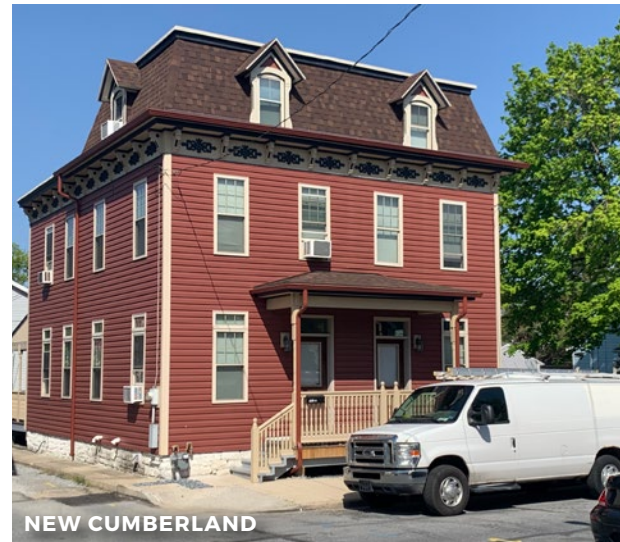
This residence does a good job of camouflaging the downspout running down the center of the façade by painting it the same color as the siding.
