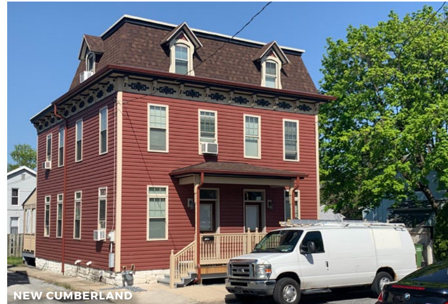
Stone foundations for frame buildings is typical.
