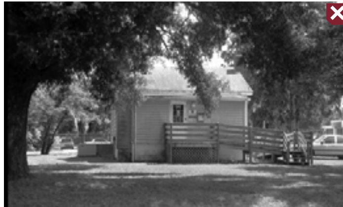
This handicapped ramp is inappropriate because it dominates the small building. The enclosure of the front porch also would not meet the guidelines.
