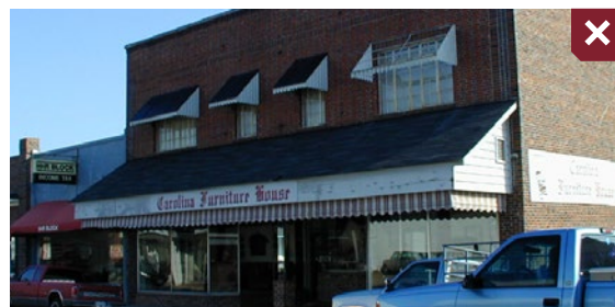
This shingled canopy conceals transom, sign panel, & upper façade components.
