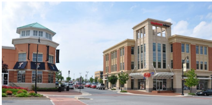
Canvas awnings (left) and metal canopies (right) on these two new commercial buildings illustrate appropriate awning treatments that respond to the windows, doors, and associated architectural forms.
